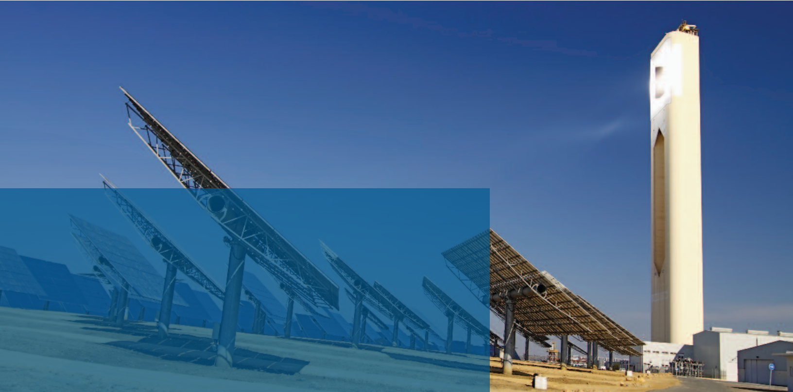
Concentrated solar power plant. © shutterstock.
